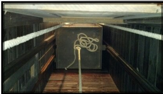
Dumbwaiter shaft as seen from above.
